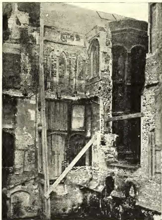
VIEW WITHIN N.W. WING DURING DEMOLITION
